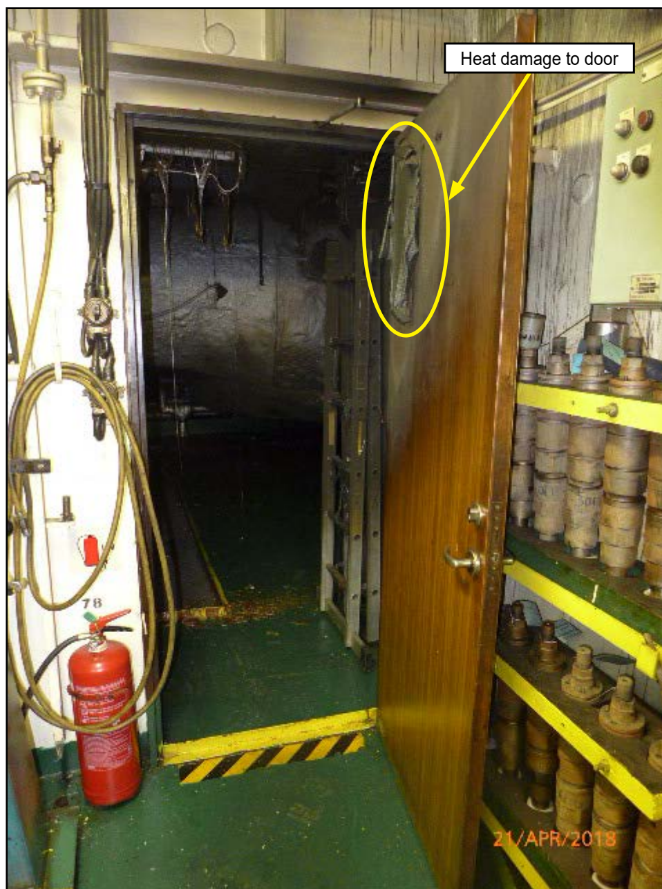
Figure 3: Purifier room door
