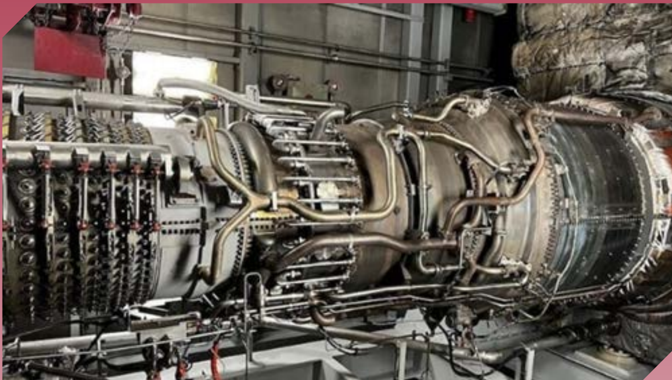
Aeroderivative turbines in ship's engine room (Photo credit: GE Power)
