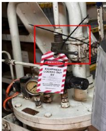
Case 2: No mechanical valve lock out was applied on the equipment
