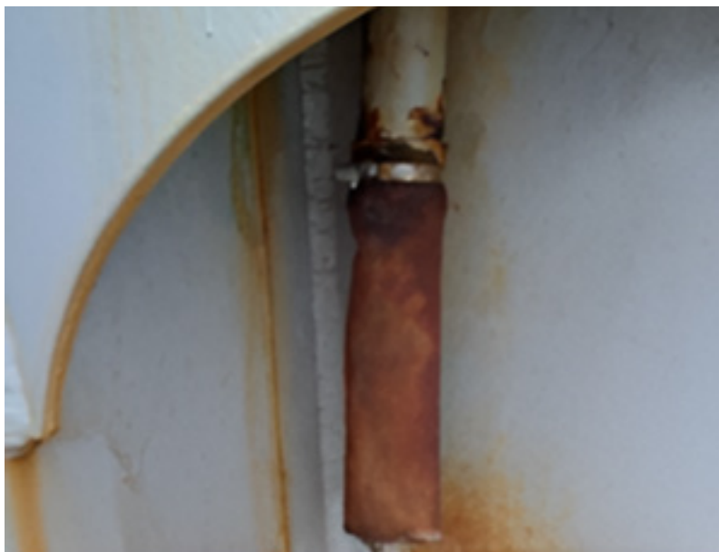
Figure 22 Non return valve temporary patch work
