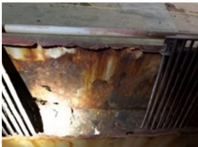
Figure 9.1 Corroded grating/deck
