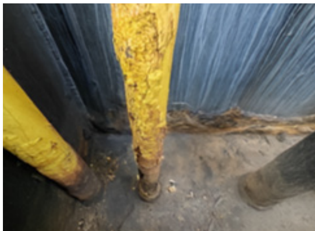
Figure 9.1 Corroded grating/deck
