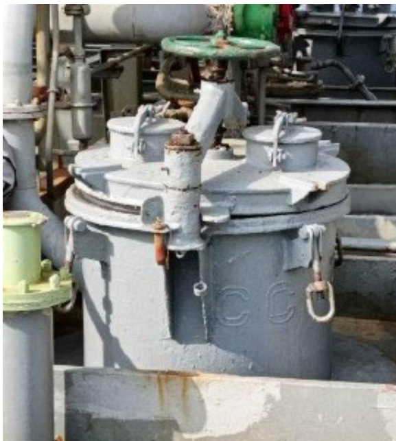
Figure 3: Photograph of a partially open cargo tank dome hatch.
