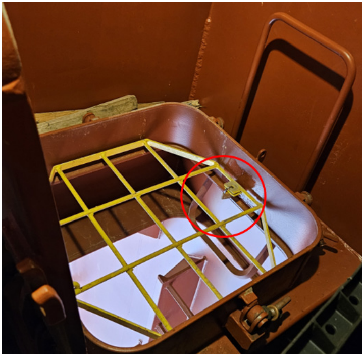
Figure 3: Secured grid (barrier) in the forward booby hatch of CH No. 1.
