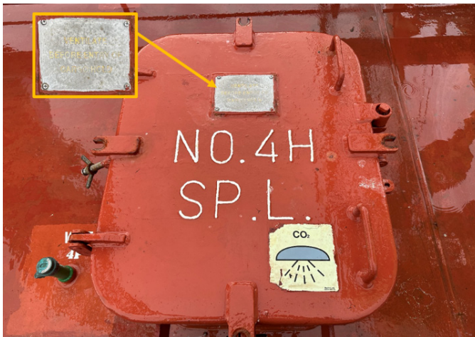
Figure 6: CH No. 4 aft access hatch cover.
